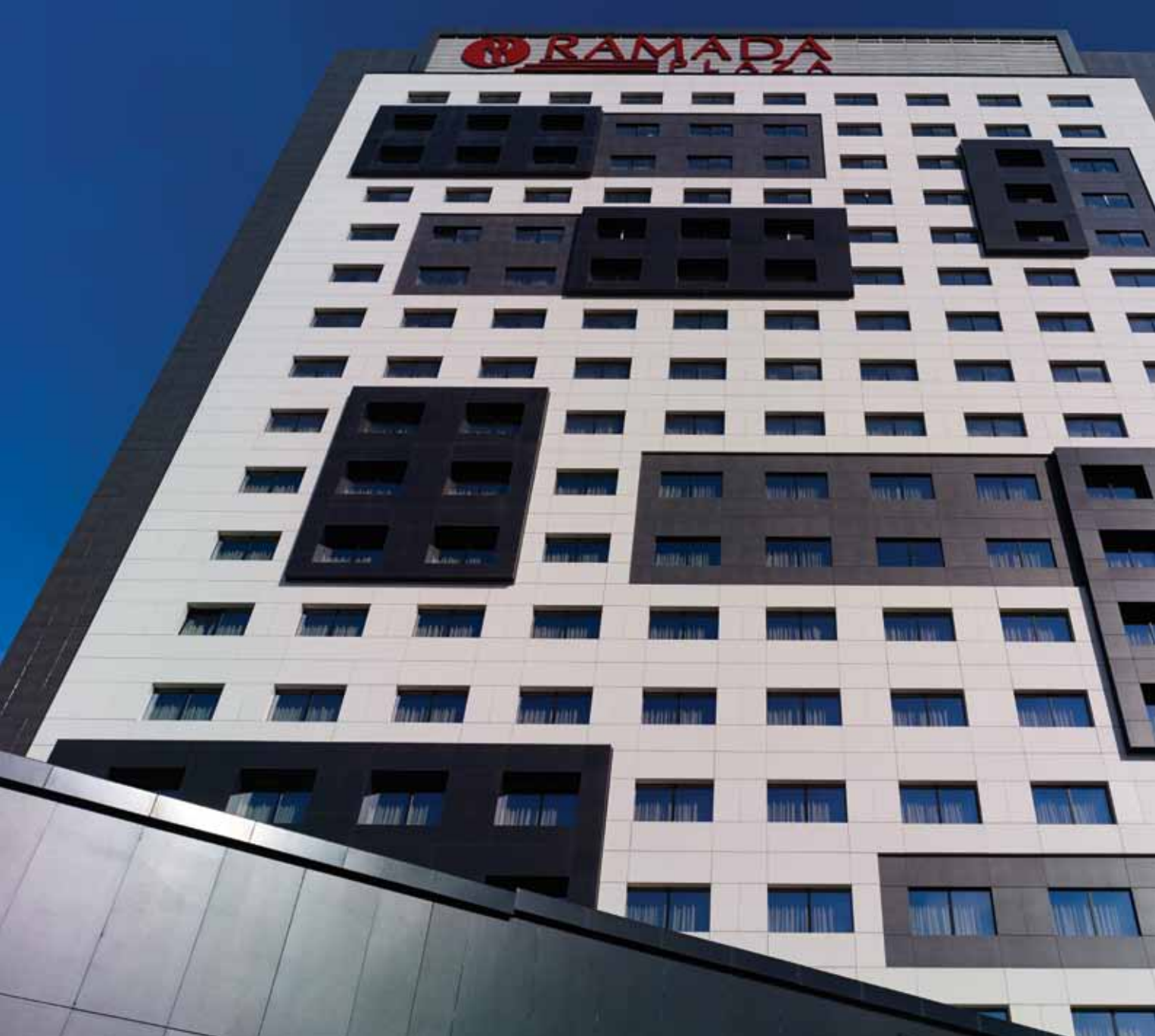
Ramada Plaza / İstanbul — Gizli Klipsli Sistem Ramada Plaza / İstanbul — Hidden Clips Fitted Facade System Mimar : M Ofis — Architect : M Office
