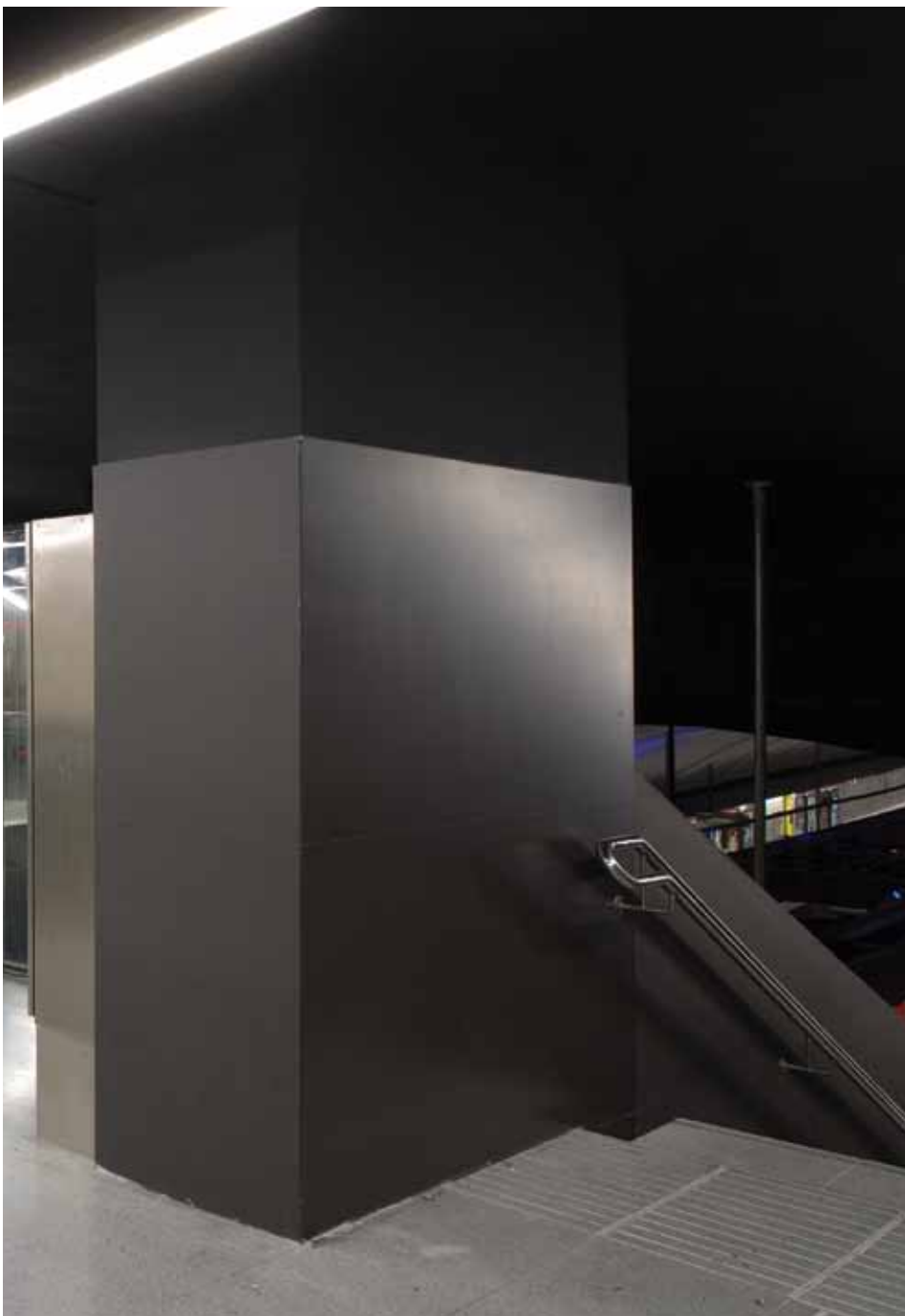
Barcelona Metro İstasyonu / İspanya — Duvar Mekanik Uygulama Barcelona Metro Station / Spain — Mechanical Wall Application
