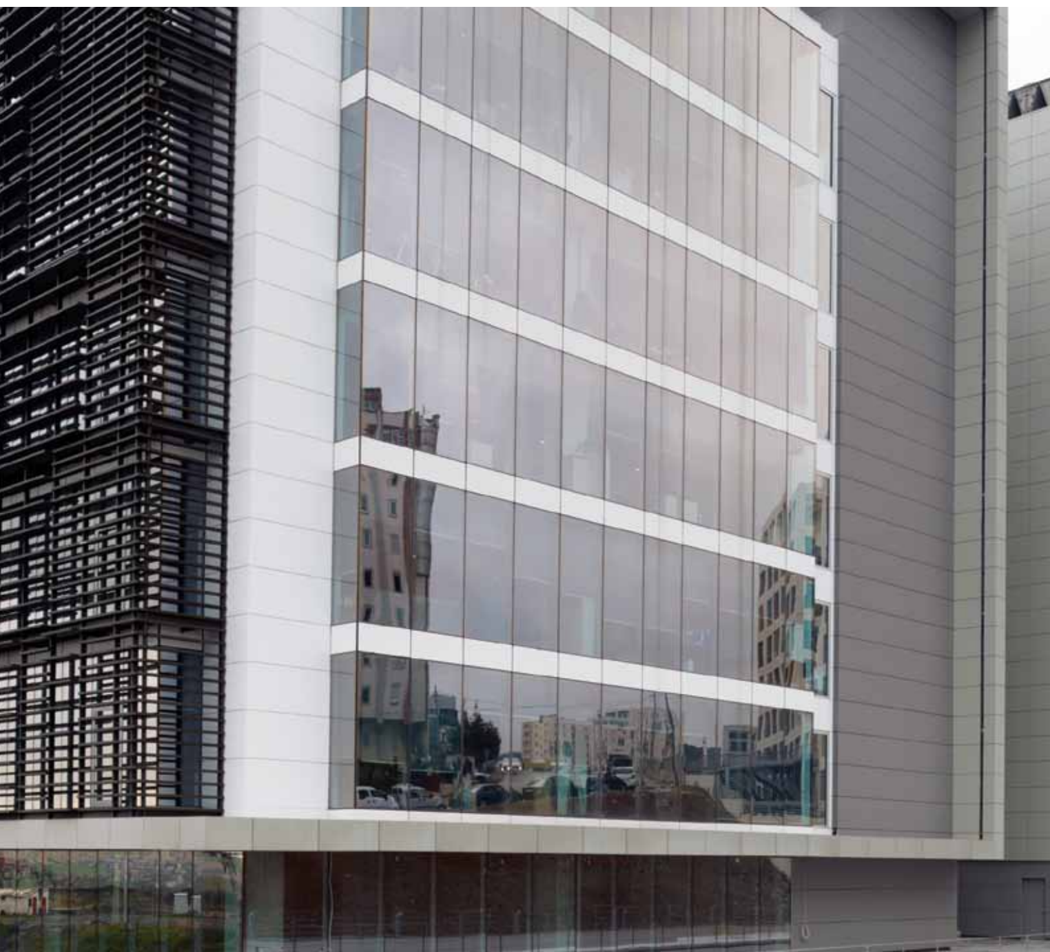
Kavaçak İş Merkezi / İstanbul — Gizli Klipsli Sistem Kavaçak Business Center / İstanbul — Hidden Clips Fitted Facade System
