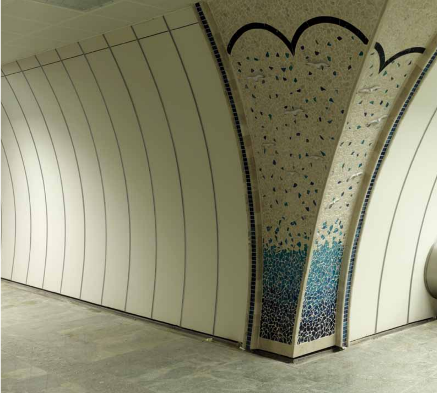
Darüşşafaka Metro İstasyonu / İstanbul — Eğrisel Mekanik Duvar Uygulama Darüşşafaka Metro Station / İstanbul — Flexible Mechanic Wall Application
