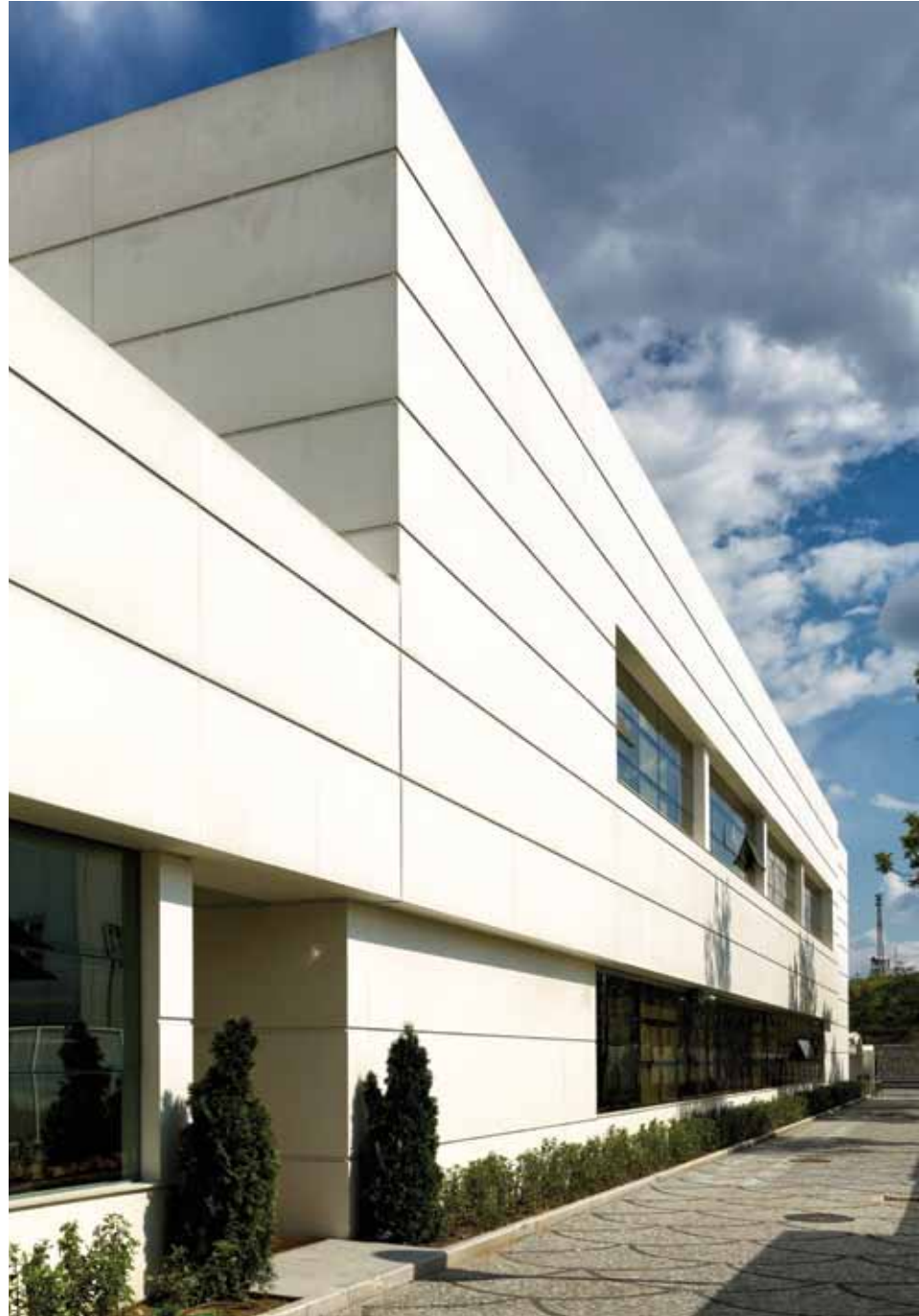
Koza Merkez Binası / Ankara — Gizli Klipsli Sistem Koza Central Building / Ankara — Hidden Clips Fitted Facade System Mimar : Promer Mimarlık — Architect : Promer Architectural Office
