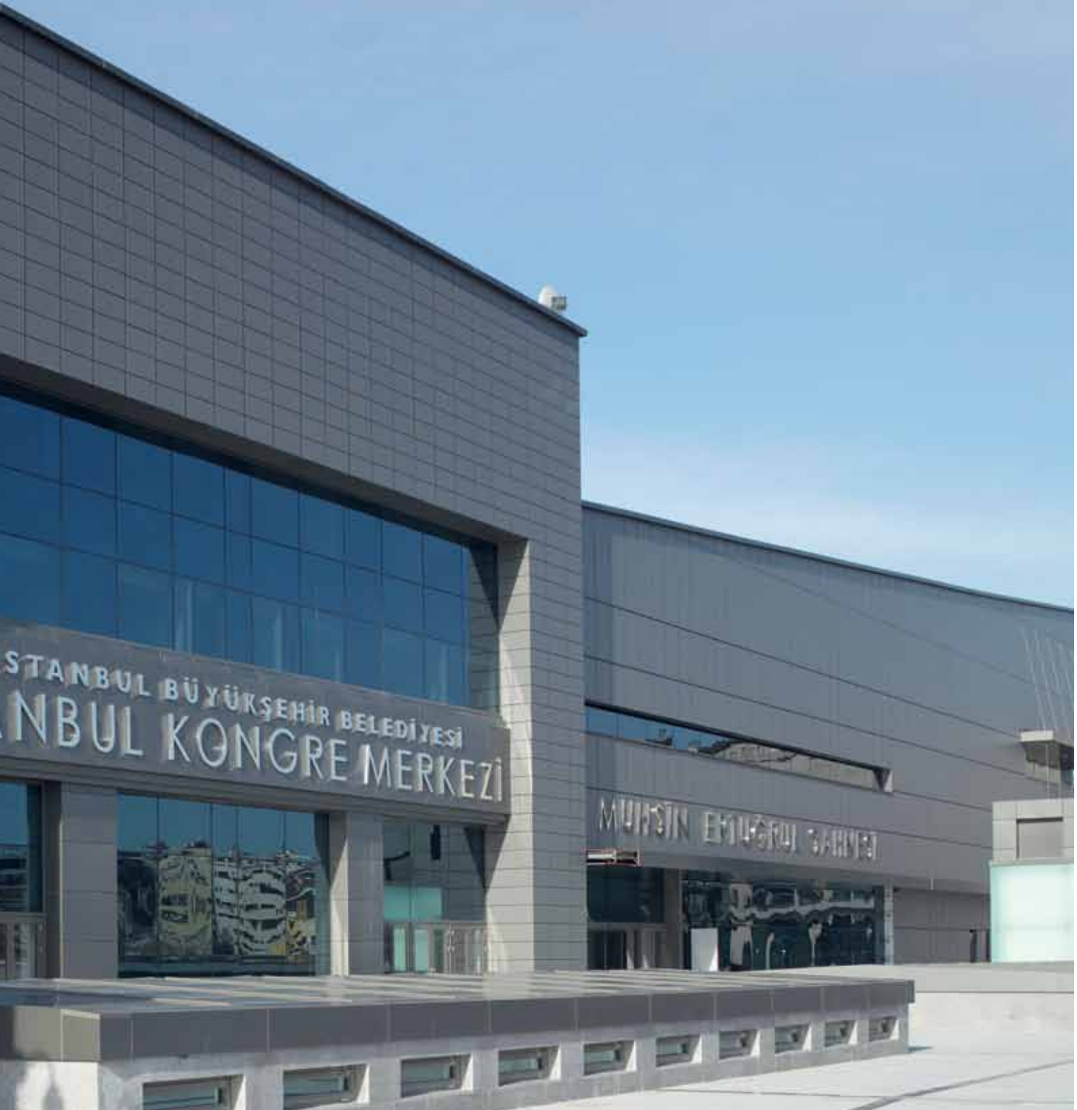
Lütfi Kırdar Kongre Merkezi, İstanbul — Gizli Klipsli Sistem Lütfi Kırdar Convention Center, İstanbul — Hidden Clips Fitted Facade System
