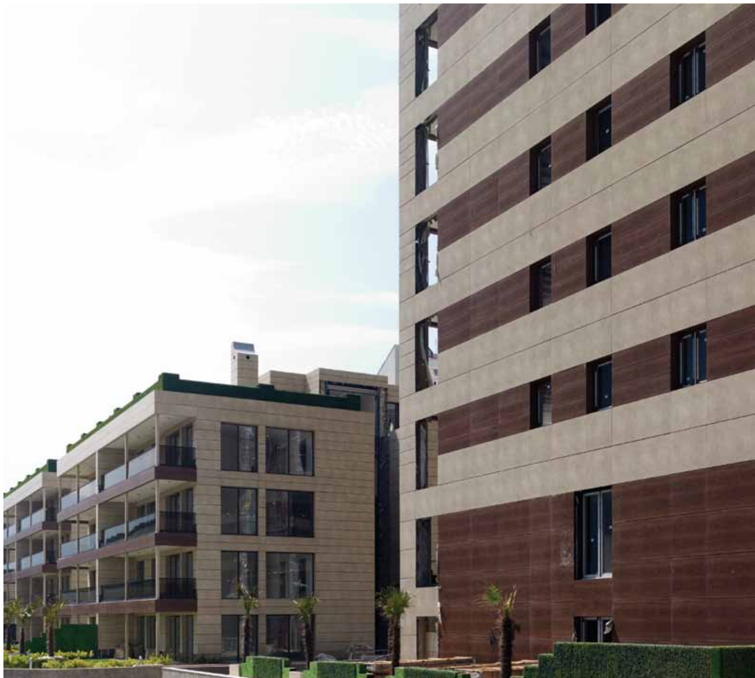
Misia Konutları, Bursa — Gizli Klipsli Sistem Misia Residence, Bursa — Hidden Clips Fitted Facade System Mimar — Architect: Emre Arolat Architects
